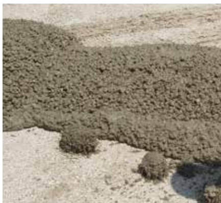
Figure 4.1.2: Fresh concrete with balling
